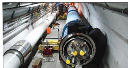
The 1000th cryomagnet during installation in the LHC tunnel on 5 September.
